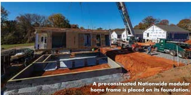
A pre-constructed Nationwide modular home frame is placed on its foundation.
